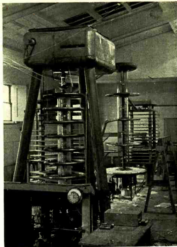
400-k.v. system with useful load in foreground as first built at the State University of Iowa. Framework in left corner is covered with lead to protect observer from X-rays.
