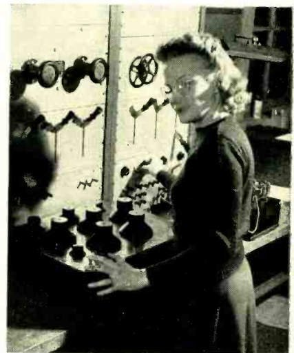
Irene Mele calibrating a standard resistance box at the Kearny Works of the Western Electric Company.
